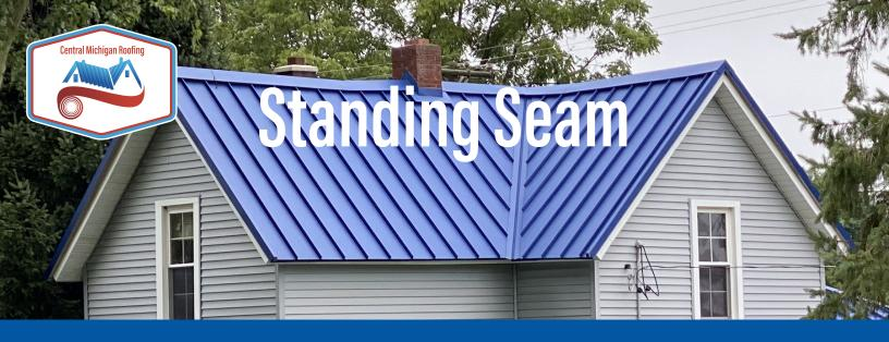
Standing Seam Metal Roofing Panels are ideal for both the residential or commercial application. Available in 34 colors and textures in 26 gauge steel, it is specifically designed so that fasteners are hidden. The end result is not only a beautiful roof, but one with limited possibility for leaks. The trim and flashing available with a standing seam roofing system are also specially designed to minimize the need of exposed fasteners.
